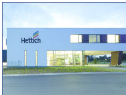
3 Compact CHP units GG 50 Furniture parts production, Hettich, Kirchlegern
