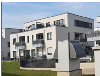
Compact CHP unit GG 50 6VRSB with air/water heat pump
