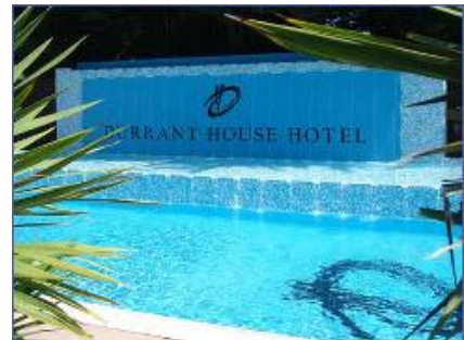
BHKW-Kompaktmodul GG 50 Durrant House Hotel, UK-Northam
