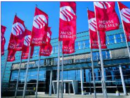
Compact CHP unit GG 50 MESSE BREMEN fairground
