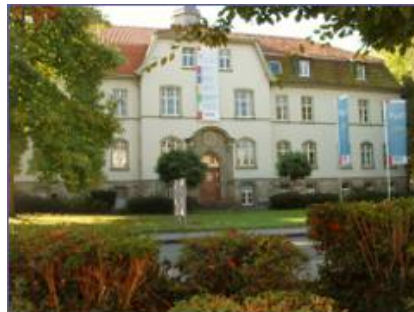
2 Compact CHP units GG 140 LWL-Klinik Lippstadt
