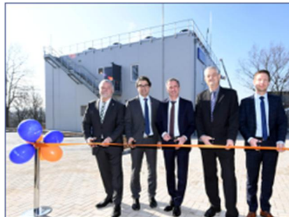
Compact CHP unit GG 330 + GG 260 EnBW combined energy center Waldbronn Contracting Award 2018
