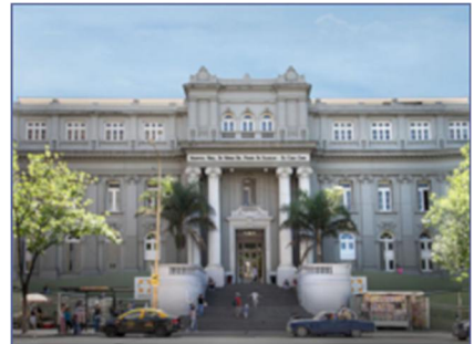
Compact CHP unit GG 50 Children's hospital, RA-Buenos Aires
