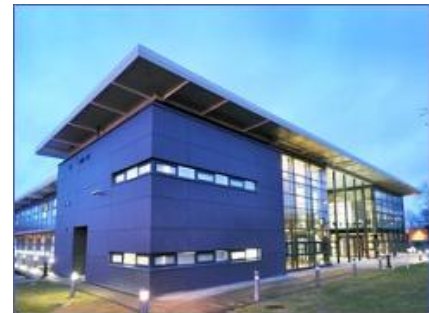
Compact CHP unit GG 50 Compact CHP unit GG 113 Cok Institute of Technology CIT, Cok (Ireland)
