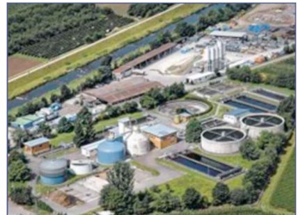
2 Compact CHP units FG 50 with emergency power function Water purification plant, Oberkirch
