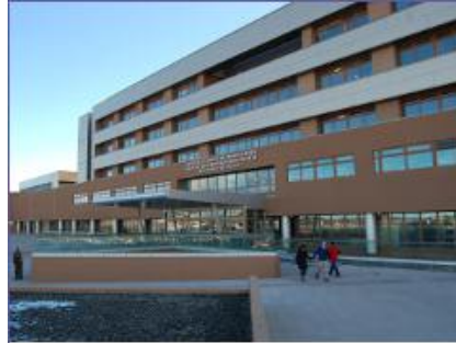
Compact CHP unit GG 402 Hospital Clinico de Magallanes Punta Arenas, Chile
