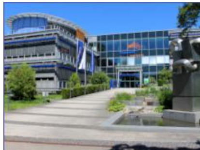
Compact CHP unit GG 70 badenova headquarters Freiburg Platin awarded by DGNB sustainable building
