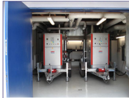
2 Compact CHP units GG 50 mobile Outdoors pool in summer and school in Winter, Enkenbach-Alsenborn
