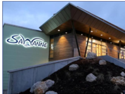
Compact CHP unit GG 50 Swimming pool & Spa SaWanne, Sangerhausen
