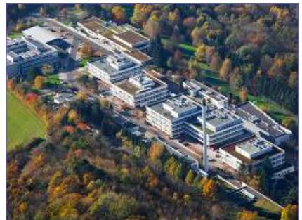
Compact CHP unit GG 402 H Compact CHP unit GG 530 Max-Planck inst. f. biophys. chemistry, Göttingen
