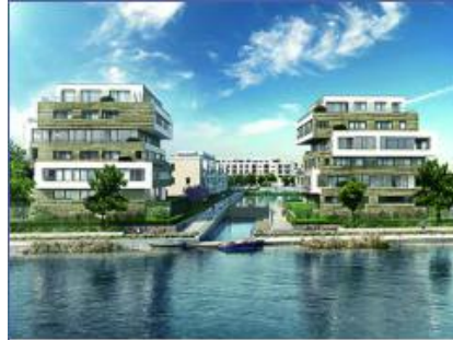
3 Compact CHP units GG 100 Housing development "52° Nord", Berlin-Grünau
