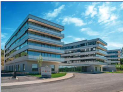
Compact CHP unit GG 100 in Container with emergency power and cooling Company HQ building "The SUMMIT", Siegen
