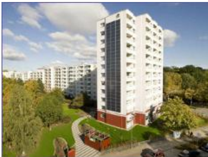
Compact CHP unit GG 140 Residential complex, Hannover-Laatzten
