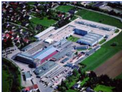
2 Compact CHP units GG 237 with emergency power function Röhm GmbH, Sontheim
