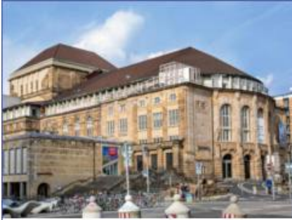
Compact CHP unit GG 330 City theatre Freiburg
