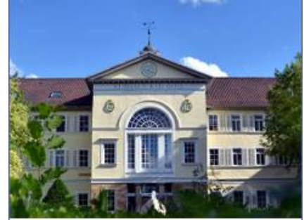
Compact CHP unit GG 237 Spa hotel, clinic and congress center Bad Boll
