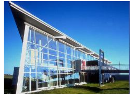
BHKW-Kompaktmodul GG 70 H with absorption chiller for climatization Multimar Wattforum, Tönning
