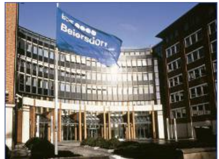
2 Compact CHP units GG 237 1 Compact CHP unit GG 140 Beiersdorf AG factories, Hamburg
