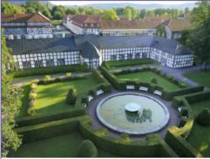
2 Compact CHP units GG 237 1 Compact CHP unit GG 140 Gräflicher Park Hotel & Spa, Bad Driburg
