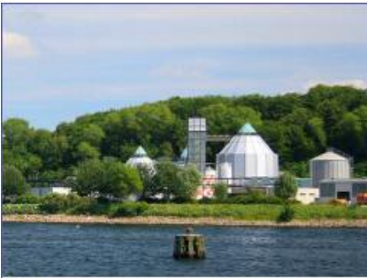
3 Compact CHP units FG 250 Water purification plant Kielseng, Flensburg
