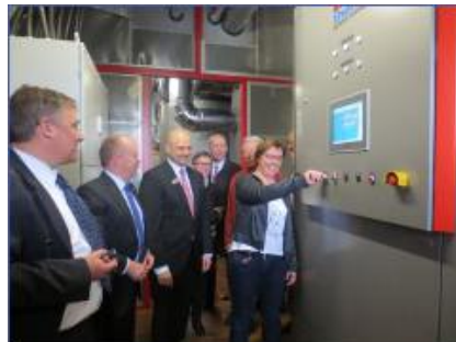
Compact CHP unit GG 530 with additional enclosure Thiebauth school Ettlingen
