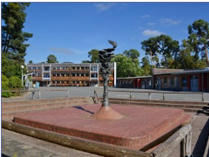
Compact CHP unit GG 50 School village Bergstrasse, Seeheim-Jugenheim
