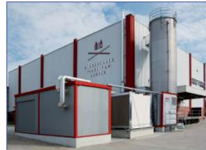
Compact CHP unit GG 402 H with hot cooling for trigeneration, container J.G. NIEDEREGGER GmbH & Co. KG, Lübeck
