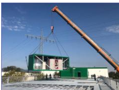
2 Compact CHP units GG 530 H with SCR catalyst, APL Landau
