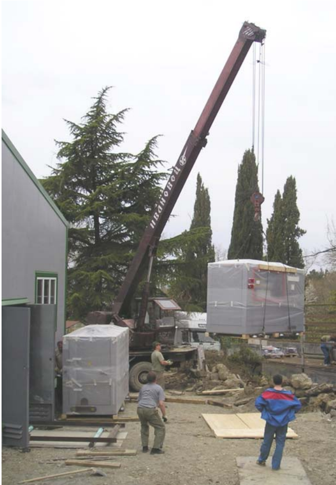
Arrival of the second (of three) CHP module GG 237 in Sochi
