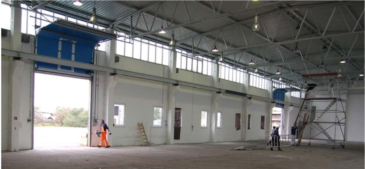
The second production hall at Nordhausen is getting ready for business.
